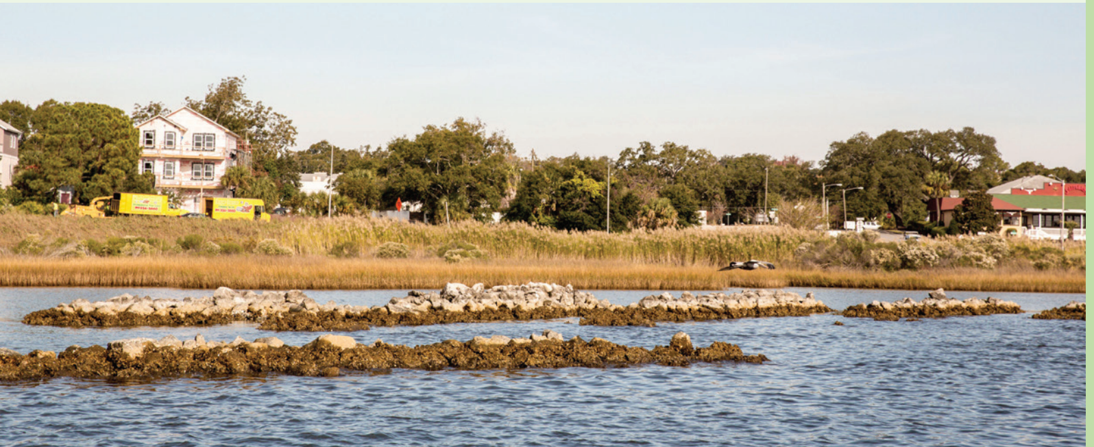
Oyster castle breakwaters protecting a vegetated shoreline from erosion. Florida Gulf Coast. Photo: Kaila Drayton/NWF.
