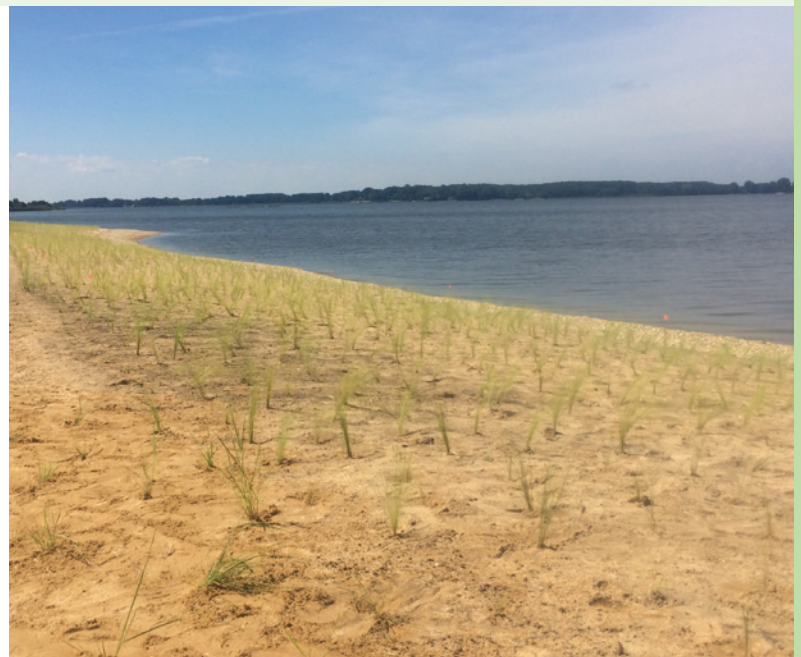
Before and after images of the Conquest Beach Living Shoreline in Maryland. The project was specifically designed to accommodate projected sea level rise. Photo: Karl Schrass/NWF.
