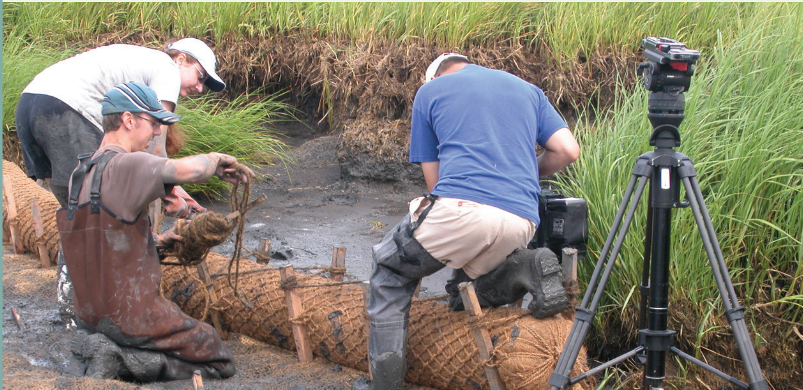
Living shoreline installation, Port Norris, NJ. Photo: PDE/Flickr.
